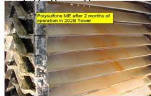
Figure 6. Polysulfone mist eliminator with polypropylene supports
